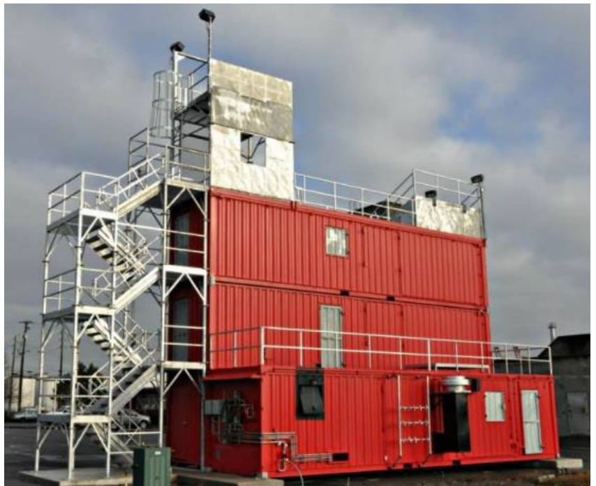
Live-Fire Training Prop – Training Center
